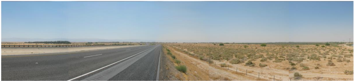
Existing setting from I-8 looking west towards the project site
